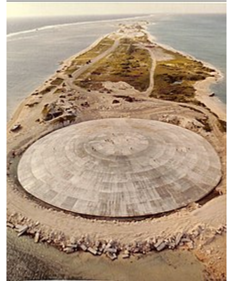
Aerial view of the Runit Dome. The dome is placed in the crater created by the " Cactus " nuclear weapons test in 1958.
